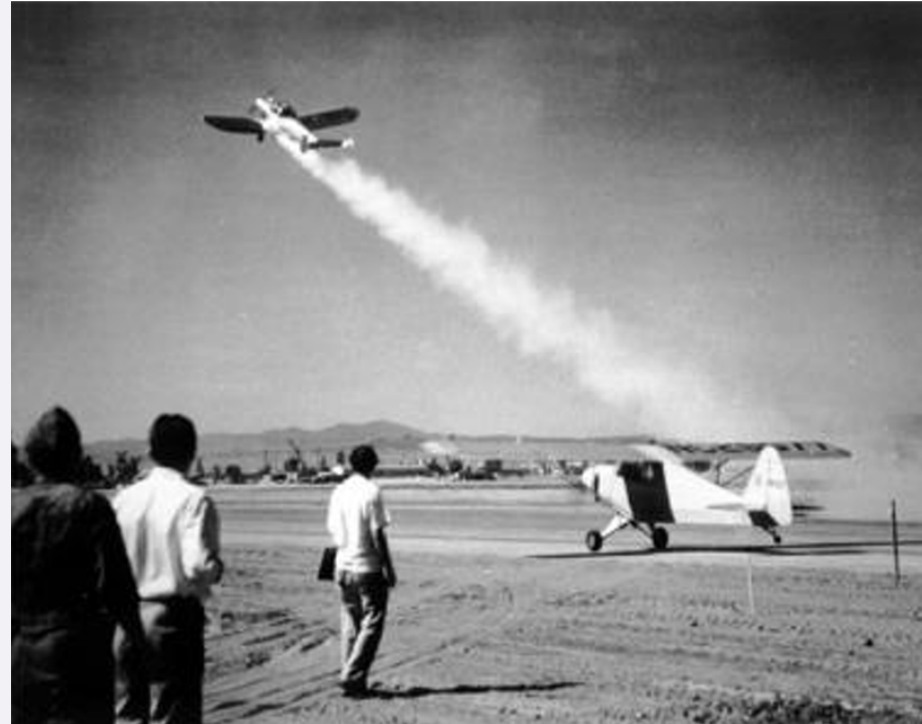
1941 demonstration of Jet Assisted Takeoff (JATO)
